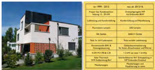
Smart-Energy-Home „Minergie-Building“ (1999), 266 m 2 EBF: TNCALL Strategy, Components and activities for the renovation are tested and measured
