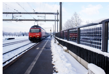
Fig 3: The world's first bifacial PV noise barrier plant on a railway line in Münsingen near Bern with a nominal power of 7.25 kWp.
