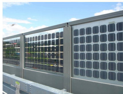
Fig 2: bifacial PV modules in Aubrugg after the refit 2005. Different glass surfaces have been used.
