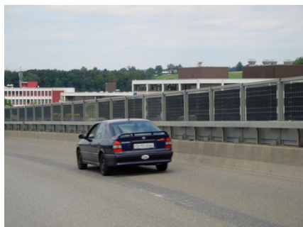
Fig 1: The original bifacial PV noise barrier built 1997 with a nominal power of 5.96 kWp.
